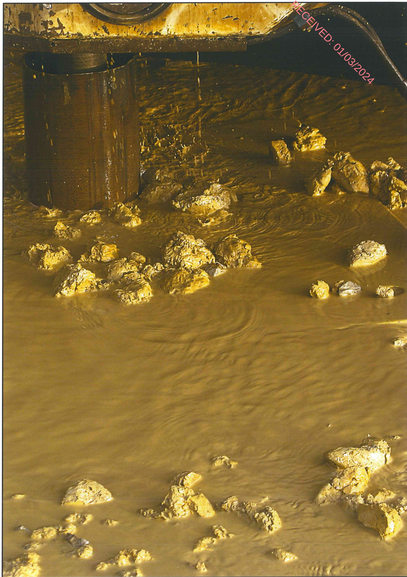
Figure 2.28 Rathcore Quarry - Large pieces of hard clay lifted during drilling borehole 3 from cavities found 37 metres below the quarry floor at the northern end of the quarry
