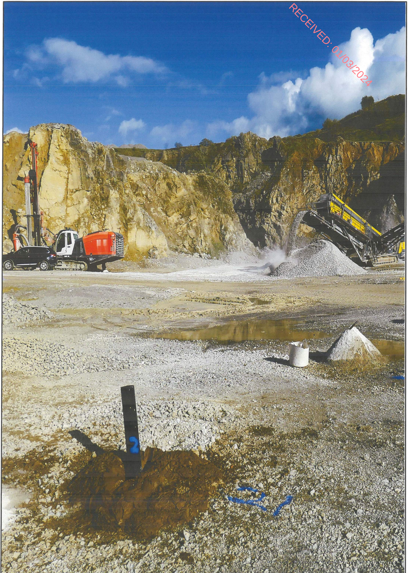
Figure 2.25 Rathcore Quarry Exploration Borehole 2, Exploration drilling rig and crusher
