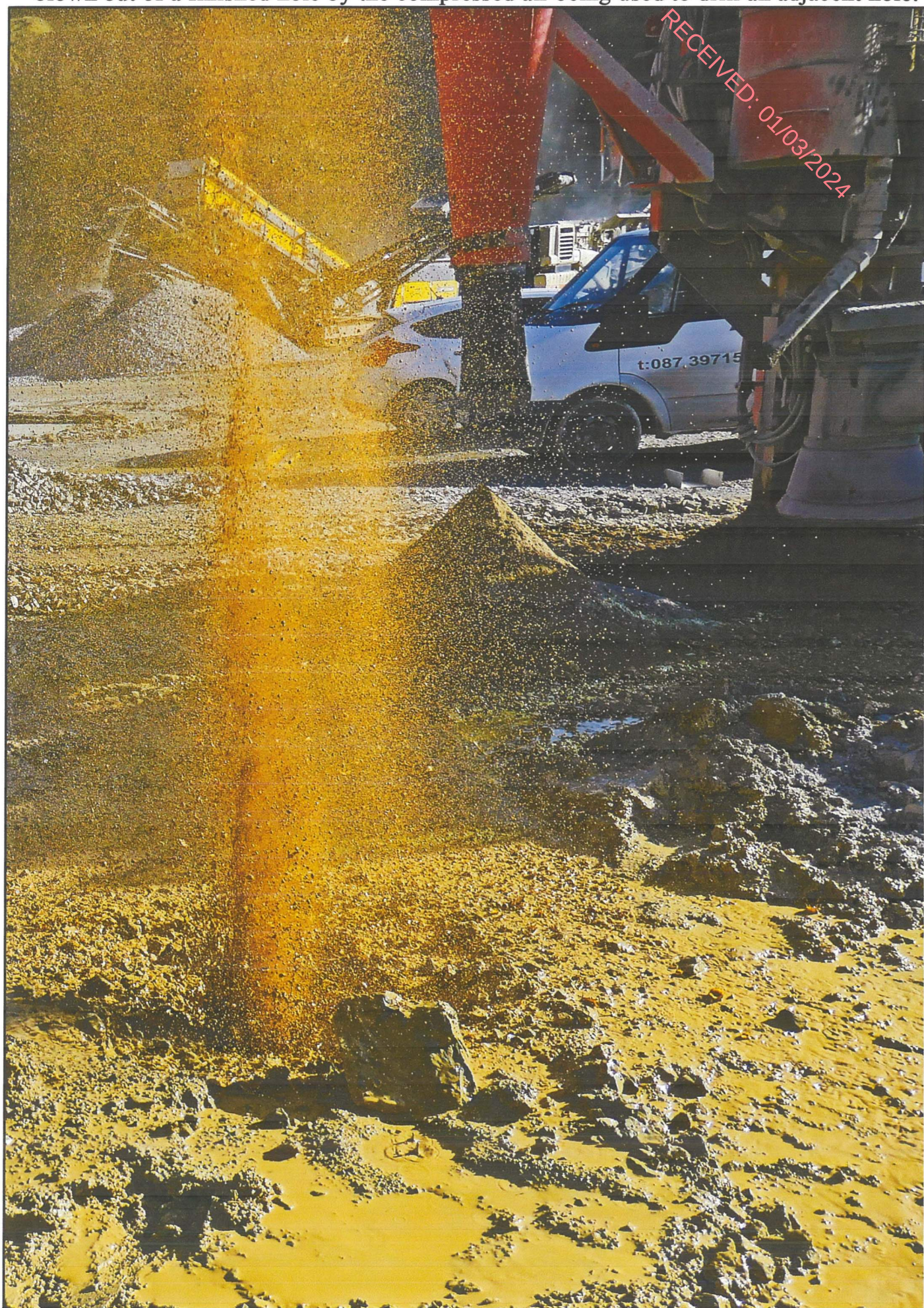
Figure 2.26 Karst conduits revealed during exploration drilling - water and clay being blown out of a finished hole by the compressed air being used to drill an adjacent hole.
